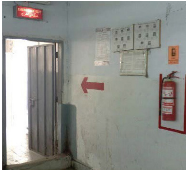
Photo of an open fire safety exit at Ali Enterprises posted by the auditing firm, RINA, on its website ( http://www.rina.org/ ). Another auditor told ILRF that the factory's fire safety exit was opened for auditors, but otherwise locked, with a guard posted in front. Photo: RINA
